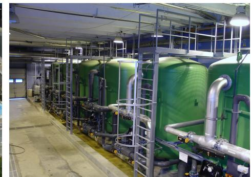
**Water processing for consumption.** We analyze and use the process most adapted according to the supply, the water level and available pressures: Decalcification, coagulation, flocculation, filtration of sand, filters activated of coal, disinfection by means of chemical agents or ozone, sterilization, desalinization by inverse osmosis, among others ways.
